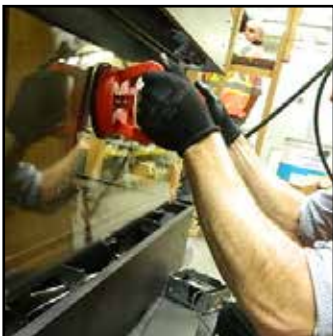
Handle glass with supplied vacuum clamps
